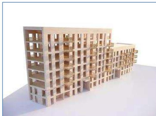
**Figure 1:** Bridport House CLT structural frame (<http://www.ttjonline.com>)
