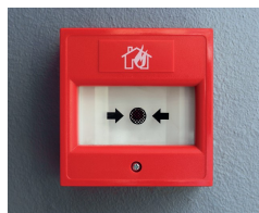
Fire alarm call point
