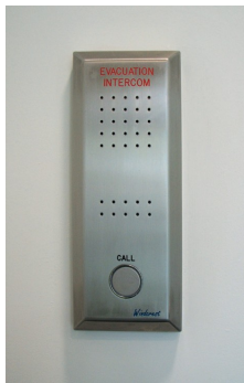
Windcrest refuge and lift communications intercom
