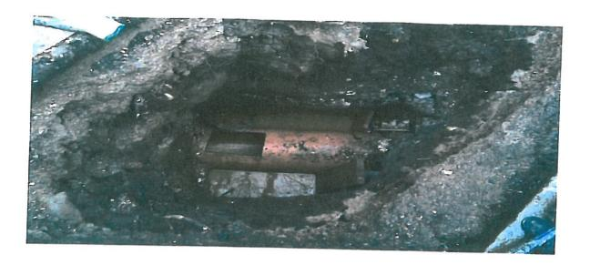
Access was cut into the drain (above) to free a blockage. The debris shown below is a tree root that was blocking approximately 50% of the bore of the drain. This section of drain was repaired with concrete and lined.
