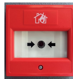
Fire alarm break glass call point
