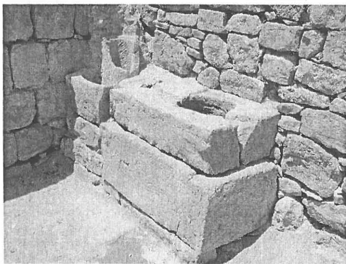
Fig. 4. Cistern-head and pipes channelling water into household cistern at Shivta.
