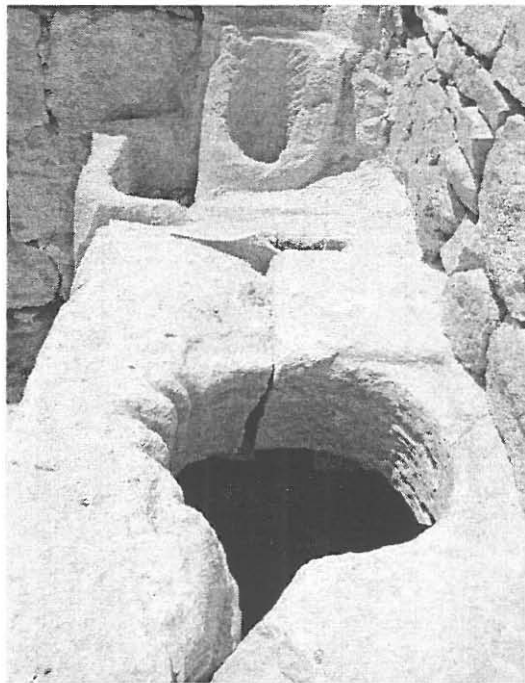
Fig. 5. Cistern-head, showing rope-marks.
